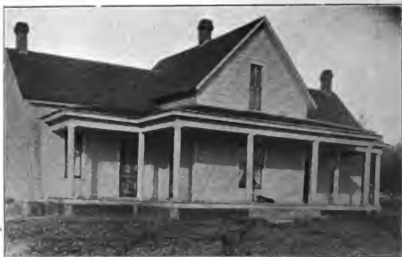
Residence of Edward P. Homes, 4 miles northeast of La Plata
